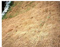
Geotextile mats not only protect ground surfaces from wind and storm water erosion but also allow vegetative growth (Source: Rolanka International, 2000)
