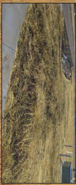
Proper amendment, seeding, and straw mulch crimping will allow this...
