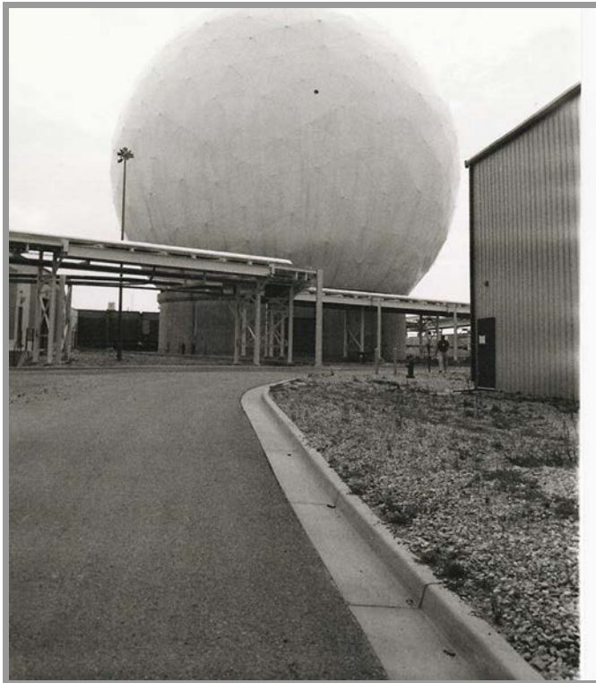
Building 404 to East
